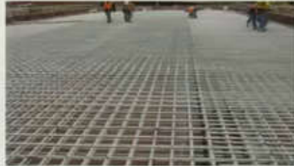
GFRP rebar used for making pedestrian bridges
